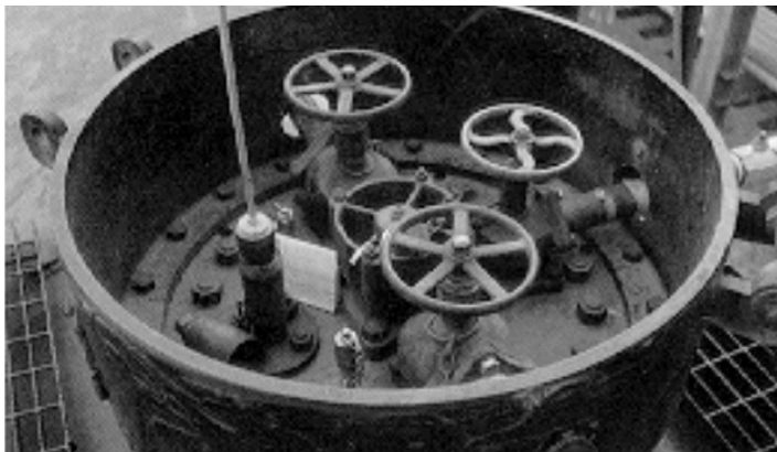
Close-up of typical LPG tank car dome, showing liquid and vapor connections and magnetic level gauge.
