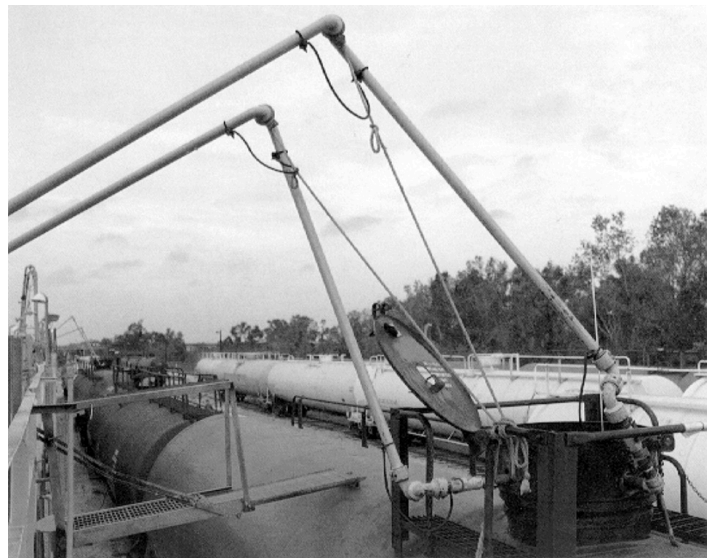
Typical butadiene rail tank car loading, showing liquid vapor connections. Magnetic gauge stick is visible.
